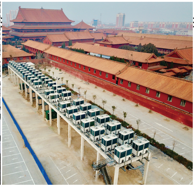
Figure 4: The “cold island” effect occurs if the air circulation around the ASHP units is not optimized. In this case, all the stations were designed as frame structures at least eight meters above the ground.
