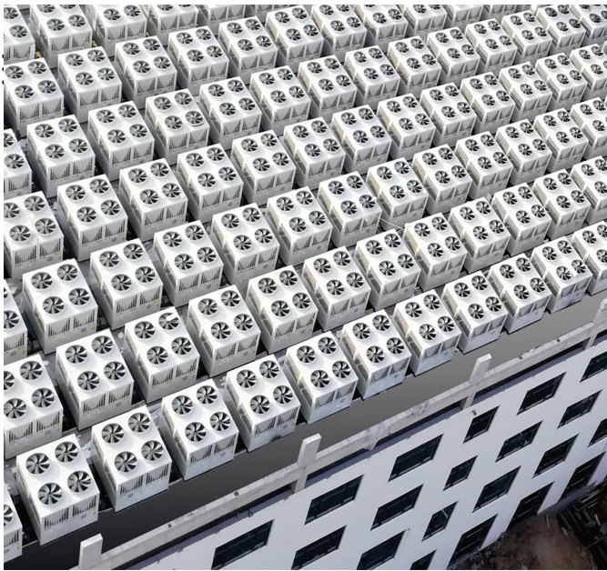
Figure 3: More than 1200 units of ASHPs were deployed as heating sources for approximately four million square meters of living spaces in large residential buildings. The challenge was how to best distribute these units and move the heat from the ASHPs to the living spaces.
